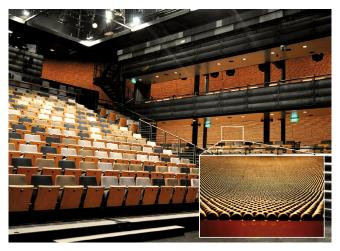
BASF's specialty foam Basotect<sup>®</sup> is fitted behind approximately 400,000 timber beads which line the curved walls of the unique oval-shaped Genexis Theatre at Fusionopolis, Singapore.
